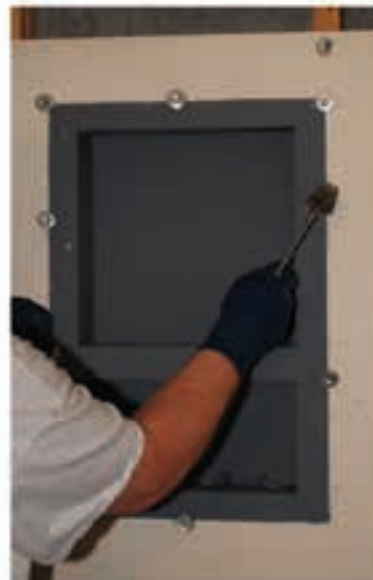
Install ProPanel ® Lightweight Backer Board or ProTEC ™ Concrete Backer Board along with a FinPan PreFormed ® Niche.
