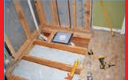
Install 2x4 blocking with top 1/4" below subfloor level. Connect drain stub to drain plate and secure.
