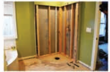
Determine shower area, remove existing subfloor.
