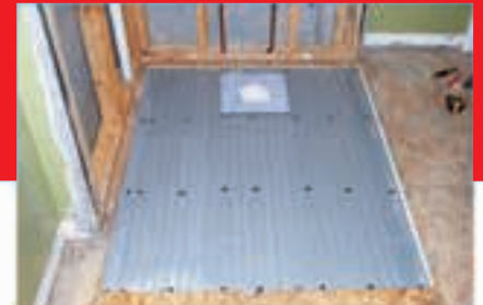
Install TI-ProBoard ® perpendicular to joists.
