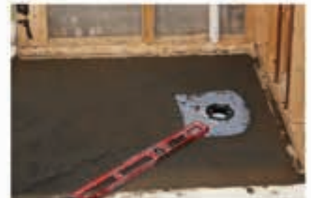
Float sloped ultra thin mud bed.
