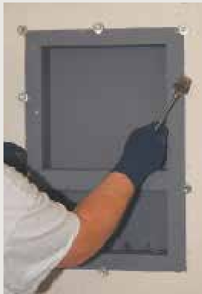
Install ProPanel ® Lightweight Backer Board or Pro TEC ™ Concrete Backer Board along with a FinPan PreFormed ® Niche.
