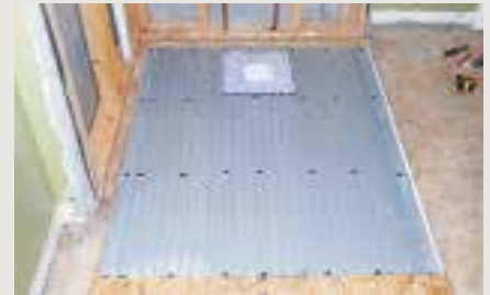
Install TI-ProBoard ® perpendicular to joists.
