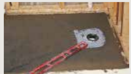
Float sloped ultra thin mud bed.
