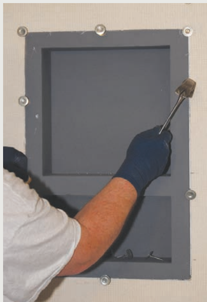
Install ProPanel ® Lightweight Backer Board or Pro TEC ™ Concrete Backer Board along with a FinPan PreFormed ® Niche.
