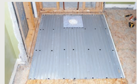
Install TI-ProBoard® perpendicular to joists.
