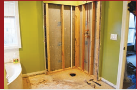
Determine shower area, remove existing subfloor.
