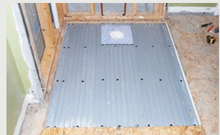
Install TI-ProBoard ® perpendicular to joists.
