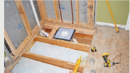
Install 2 x 4 blocking with top 1/4" below subfloor level. Connect drain stub to drain plate and secure.
