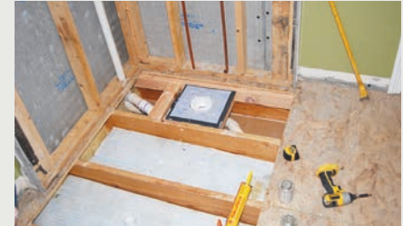
Install 2 x 4 blocking with top 1/4" below subfloor level. Connect drain stub to drain plate and secure.
