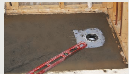
Float sloped ultra thin mud bed.
