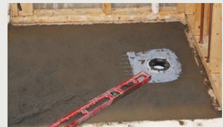
Float sloped ultra thin mud bed.
