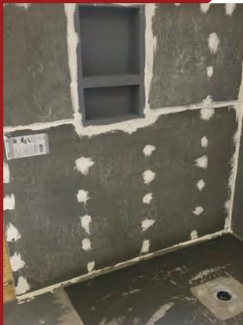
ProPanel is made of high-density expanded polystyrene insulation reinforced, on both sides, with fiberglass mesh and a polymer cement coating that offers 100% waterproof protection. It's easy to carry, cut and installs directly to framing members.
